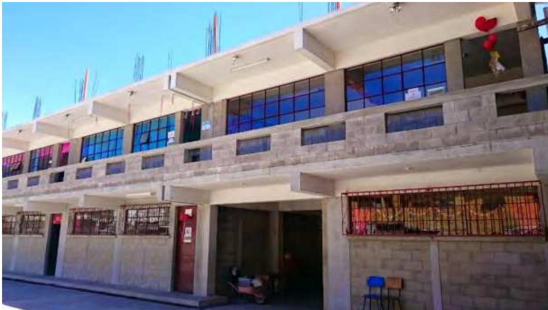
Figure 18 – New two-story confined masonry building
