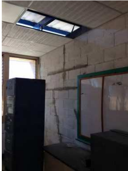
Figure 4 – Repaired wall cracks
