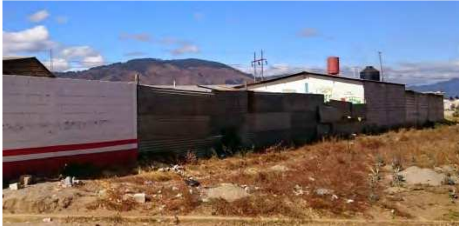
Figure 36 – Temporary perimeter wall
