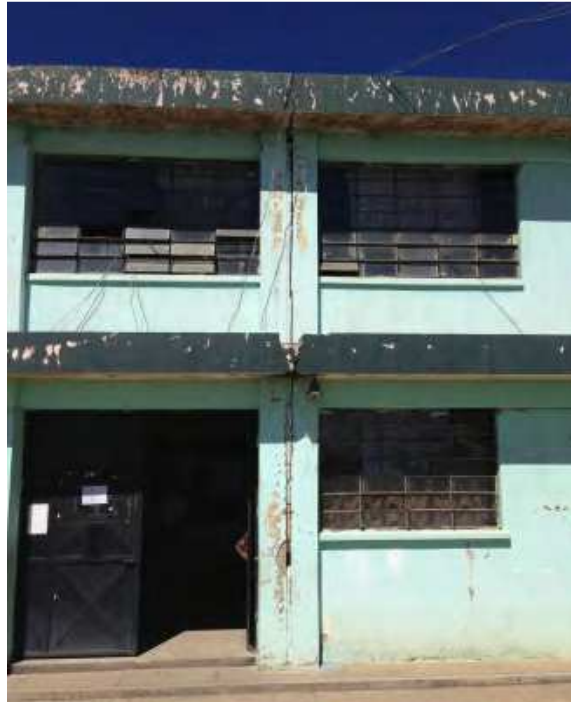
Figure 11 – Seismic joint between concrete frame buildings – mortar-covered & foam-filled
