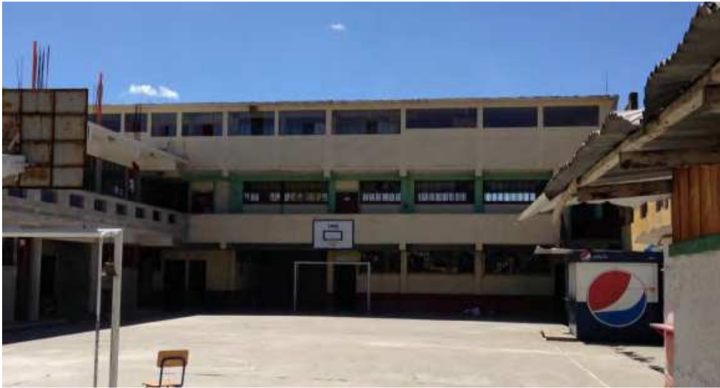
Figure 17 – Three-story confined masonry building
