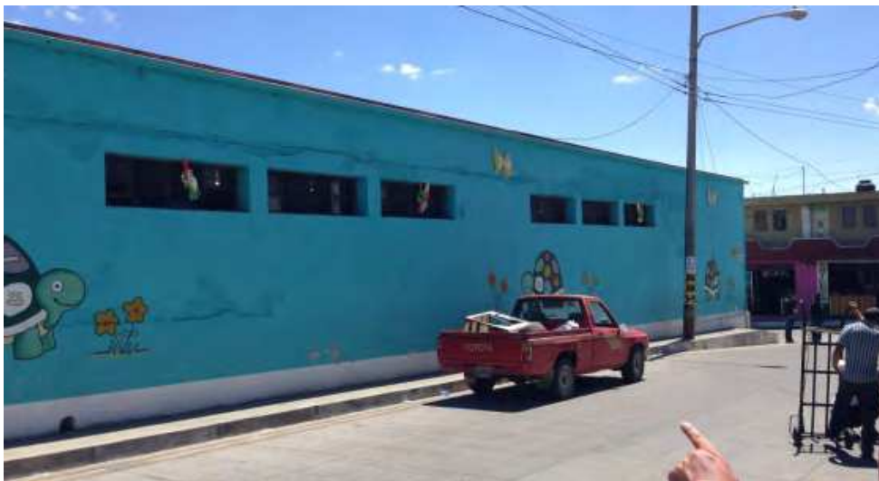
Figure 27 – Side of school along classroom wing (from exterior)
