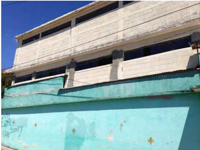
Figure 24 – Short column repairs (double columns installed)
