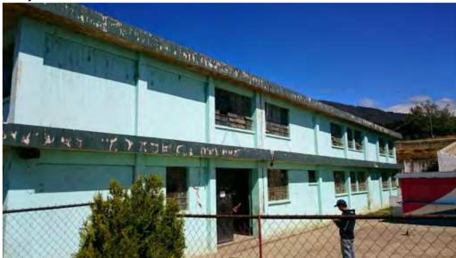
Figure 9 – Concrete moment frame building
