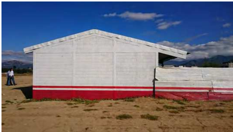
Figure 35 – Confined masonry gable end wall
