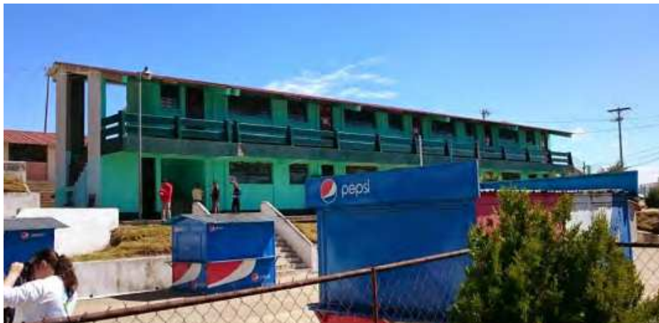
Figure 10 – Confined masonry building
