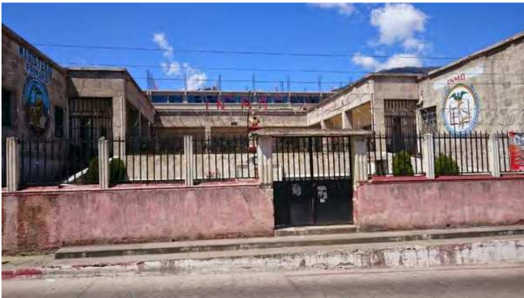
Figure 16 – Front of INMO – one story partially confined buildings
