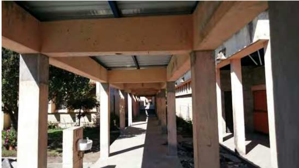
Figure 8 – Repaired concrete frame canopy structure
