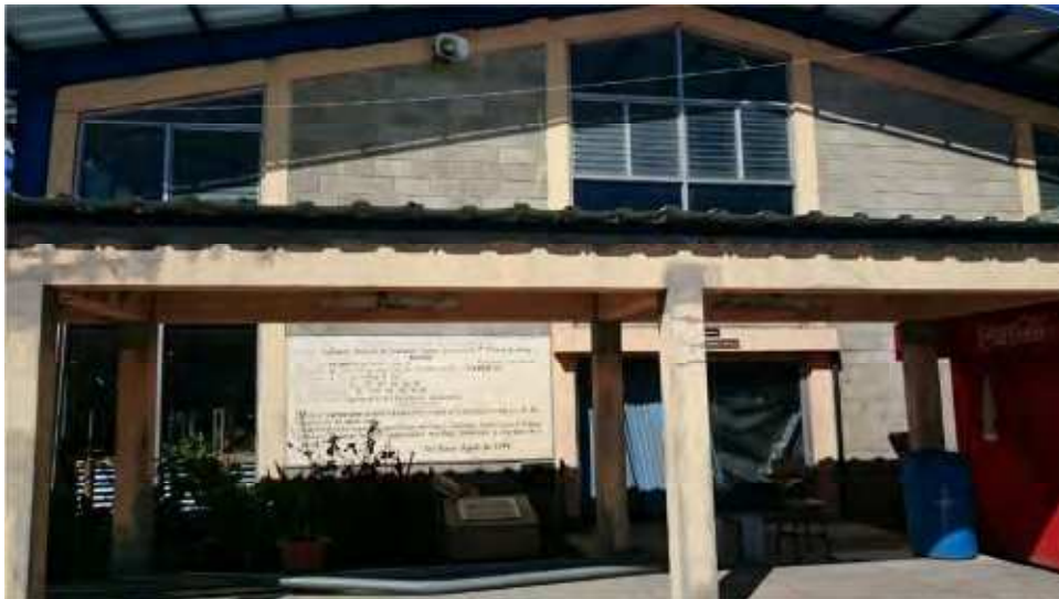
Figure 2 – Administrative two-story building
