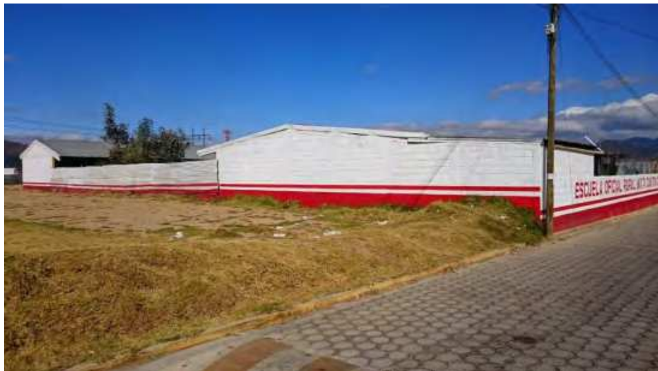
Figure 34 – Low-rise confined masonry school buildings.
