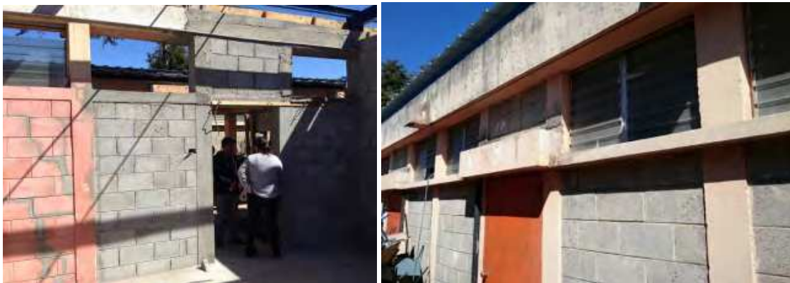
Figure 7 – Repaired short pier above door (left) and existing pier (right)
