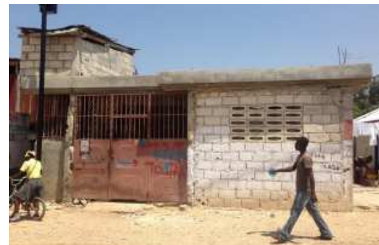
Figura 2: Typical masonry home in Port-au-Prince, Haiti
