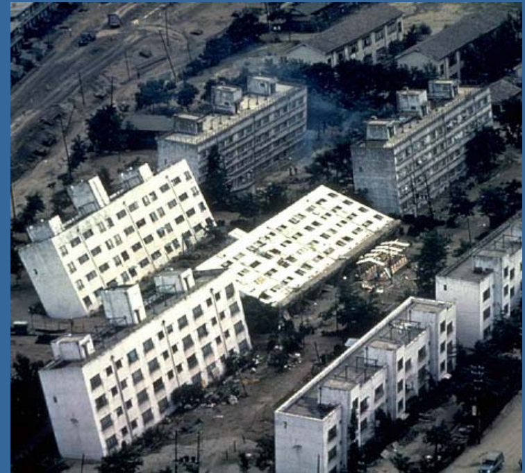
1964 Niigata, Japan Earthquake
