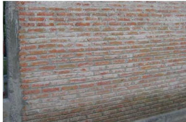
Figure 2. Well-built confined masonry wall, house on edge of heavily damaged Pleret (Bantul), S7.83686° E110.41552°, IMG_6640
