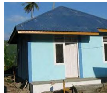
Figure 1. Build Change Pilot Project House, Hipped Roof (Owner: Rusdi Razali).
