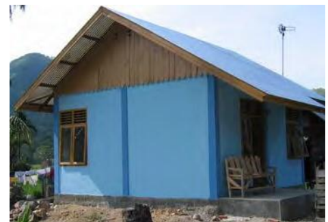
Figure 7. Build Change Pilot Project House, Pitched Roof. Owner: Ruslan AB.
