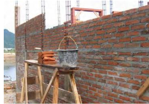
Figure 6. Wall with Horizontal Reinforcement.
