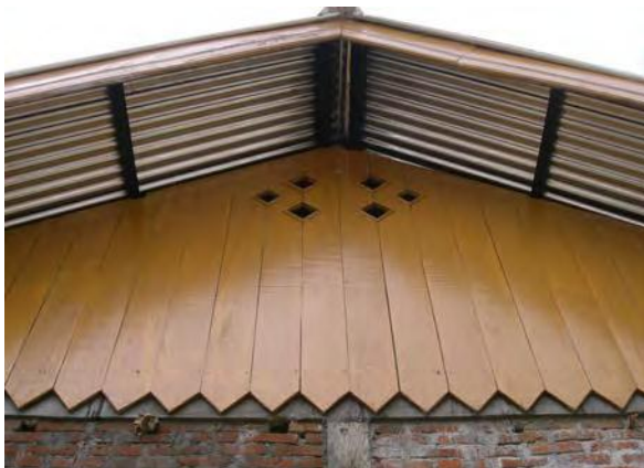
Figure 6. Papan Gable (Maimunah's house designed and built by Build Change, Keunue ue, Peukan Bada, Aceh Besar)
