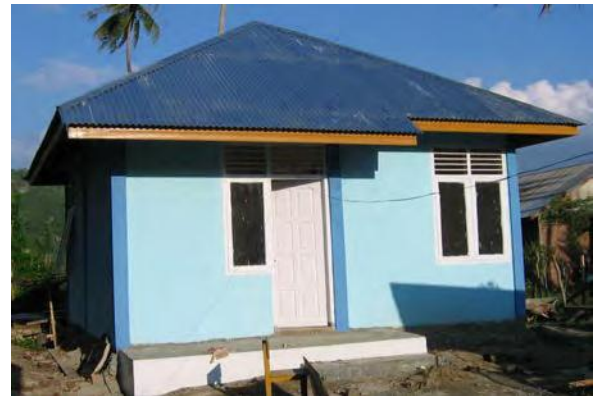
Figure 7. Rabung Empat Roof (Rusdi Razali's house designed and built by Build Change, Keunue ue, Peukan Bada, Aceh Besar)
