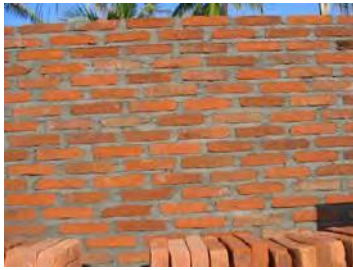
Figure 15. Typical wall built by Build Change-trained mason
