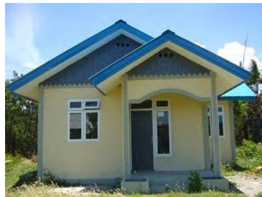
Figure 15. Covered terrace with lightweight wall, Build Change designed house for Catholic Relief Services (Aceh Besar)
