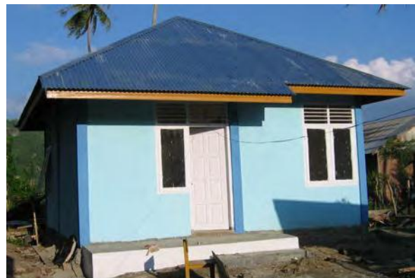
Figure 10. Rabung Empat Roof (Rusdi Razali's house designed and built by Build Change, Keunue ue, Peukan Bada, Aceh Besar)
