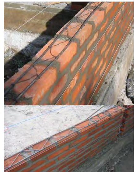
Figure 9. Horizontal reinforcement fabricated on-site with binding wire (top) and prefabricated at welding shop (bottom).
