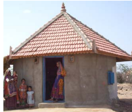
Fig. 8. Circular, stabilized earth-walled structure with pitched roof, appropriate for hot climate (Bhuj EQ)
