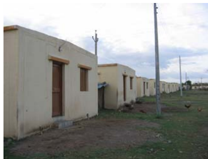
Fig. 10. Relocated village that is predominantly unoccupied due to lack of water (Killari EQ)
