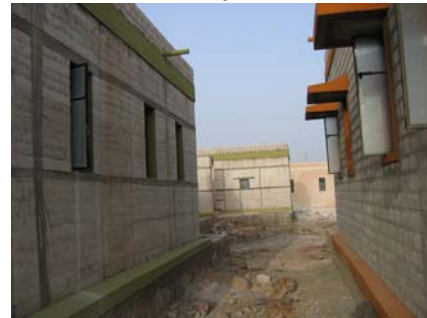
Fig. 9. Houses built early in the program without lintels (left), windows with substantial lintels built later (Bhuj EQ)
